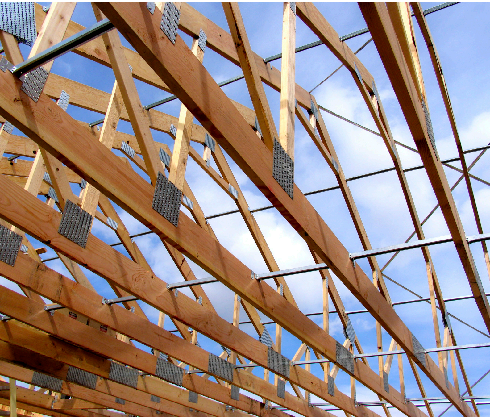
Metal connectors for Trusses
