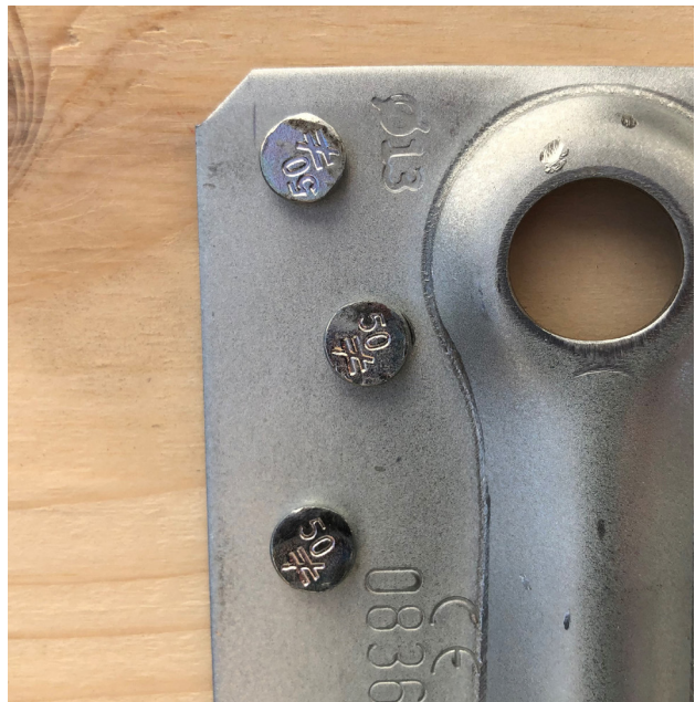
Stamps on the connectors together with the stamps on the head of the nails makes it easy to audit the installations afterwards.
